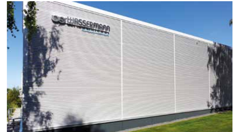
High rack storage area
